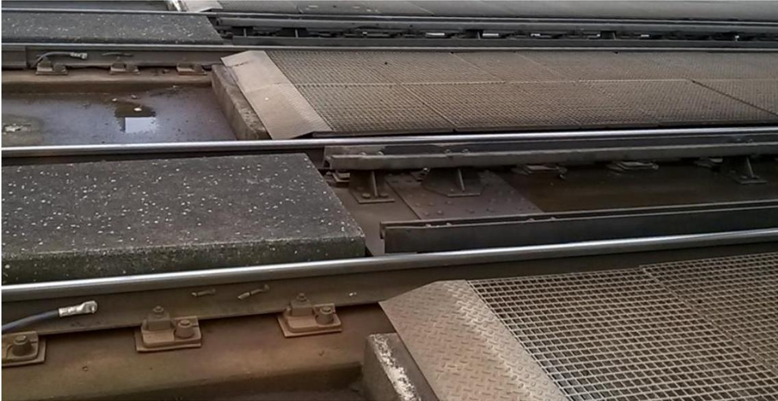
*Figure 3 Direct fastening on concrete (left) and steel parts (right) of the large bridge across the river IJssel in Deventer. Photo by Movares.*
