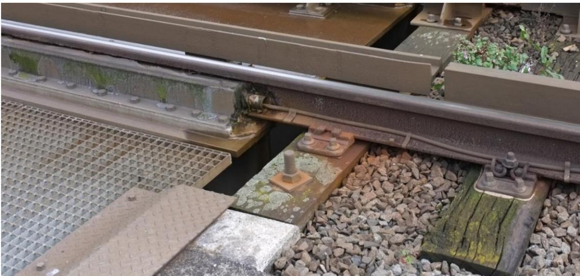
*Figure 4 Transition from embedded rail (left) to ballasted track (right) on a steel bridge across the river Roer in Roermond. Photo by Movares.*
